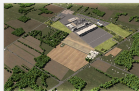
New site - under construction
